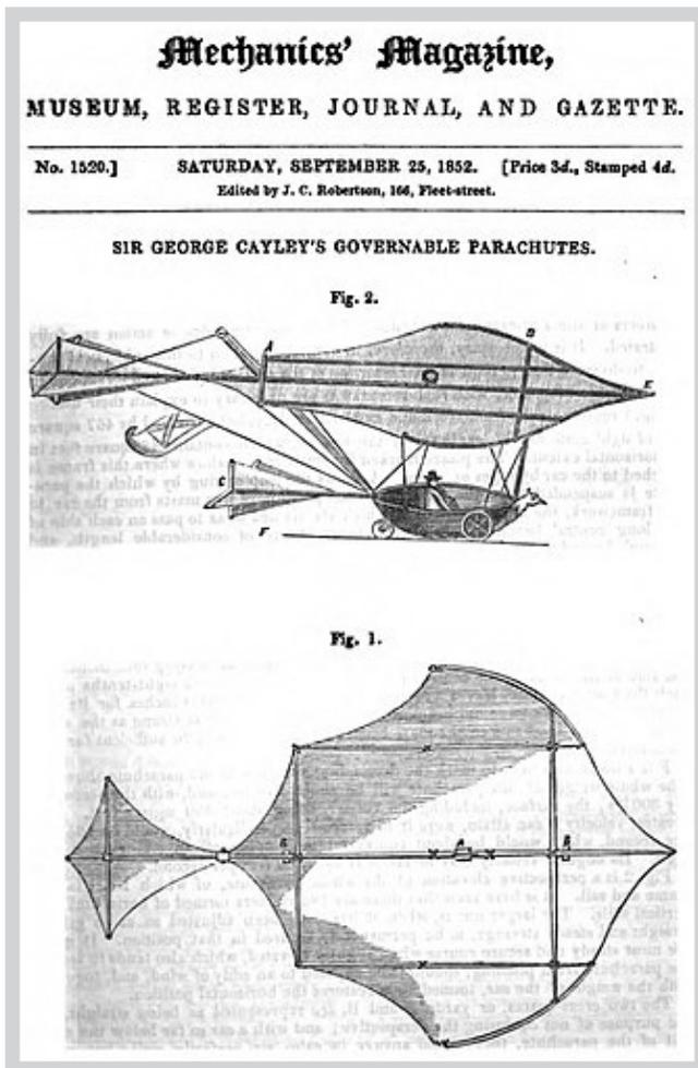
*Modern aerospace began with Sir George Cayley in 1799. Cayley proposed an aircraft with a 'fixed wing and a horizontal and vertical tail', defining characteristics of the modern airplane.*
